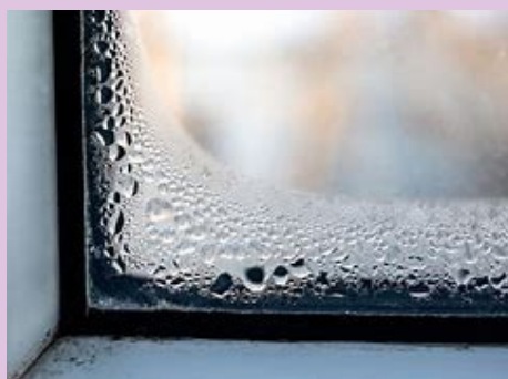
Signs of high levels of humidity that could be present in your property.
